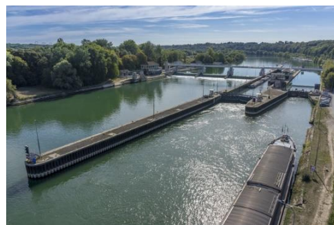
Photo / Source – ProXiti – Ecluse d'Evry
